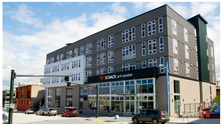
Artspace Everett Lofts, Everett, WA // Photo Credit: Artspace
